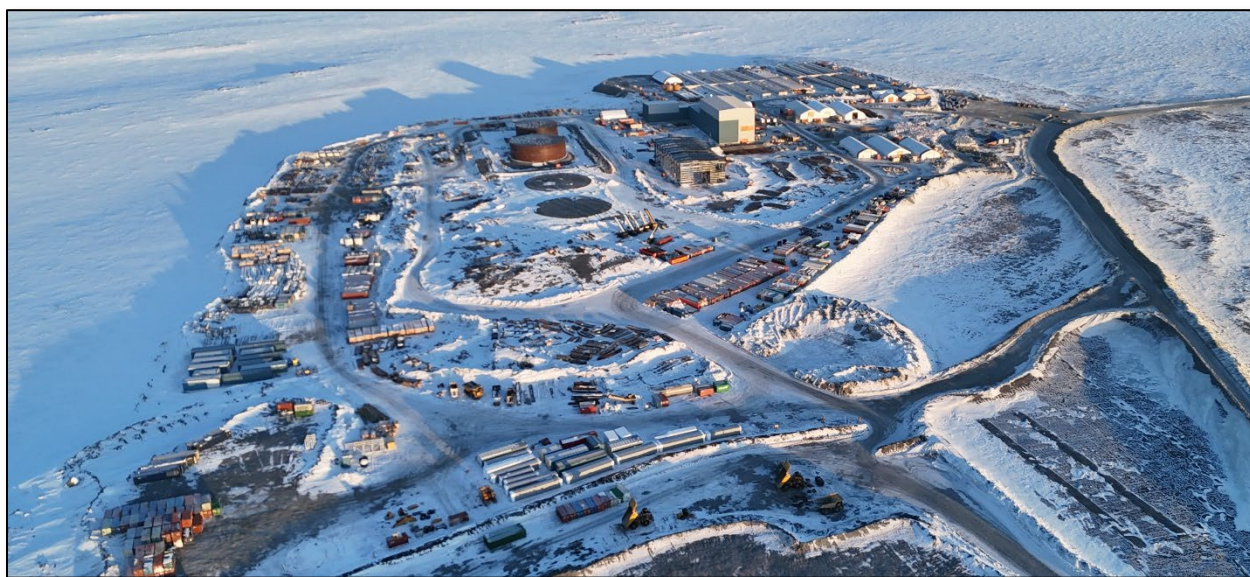
Goose Project site laydown area – April 2024
